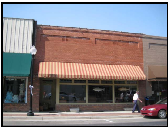
Carr Building—East Union Street
